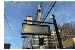
Sacramento Regional Transit Authority, USA
