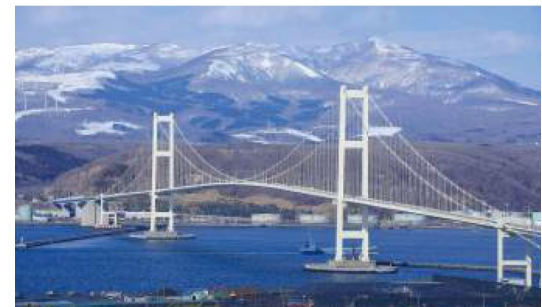
Figure 3. Hakucho Bridge [1988-1997], Chodai (Client: Ministry of Land, Infrastructure, Transport & Tourism)
