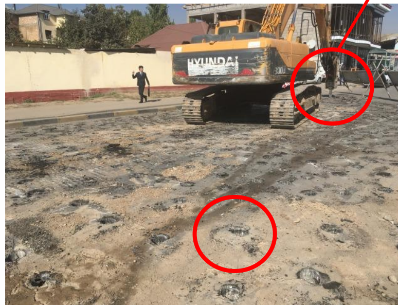
Make a hole with using a braker
