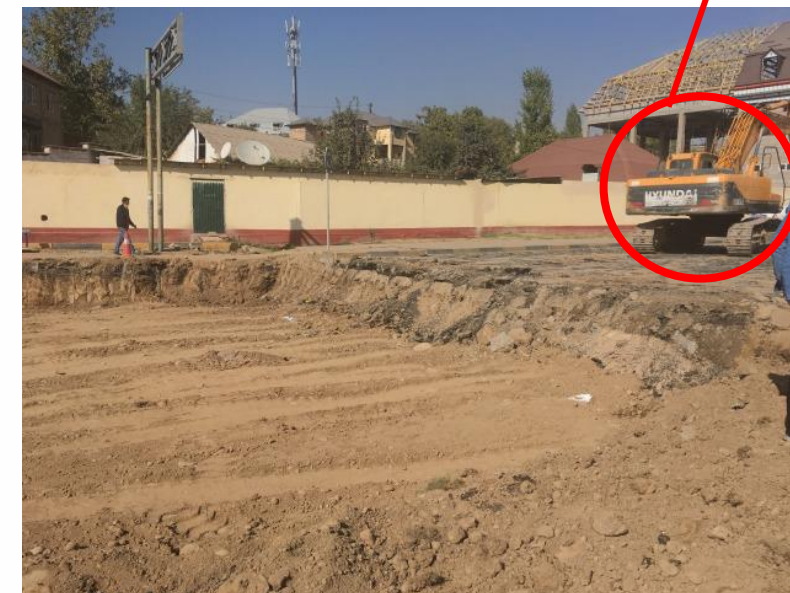
Peel off with using a excavator
