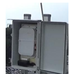
Installing access point
